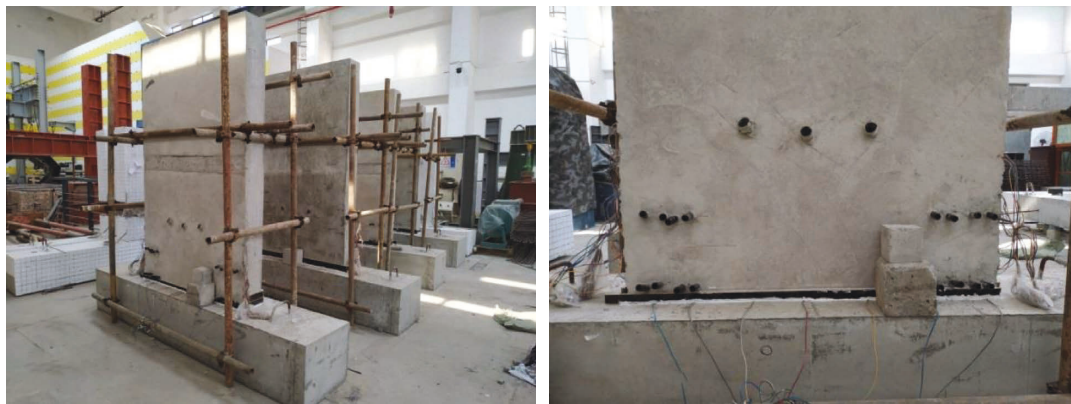
FIGURE 2: Assembly process of precast shear wall.
