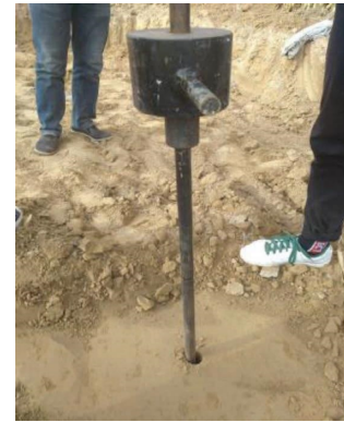
FIGURE 8: Heavy-duty penetration test.
