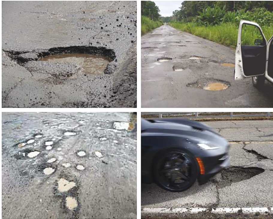
FIGURE 3: Sample of pothole images from the dataset.
