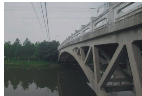
FIGURE 4: Side view of the bridge.
