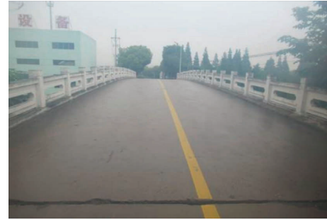
FIGURE 3: Frontage view of the bridge.
