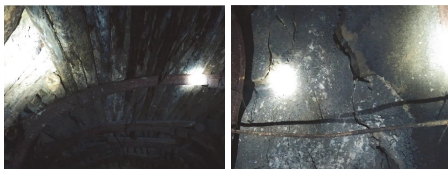
FIGURE 11: -228 m horizontal U-shaped steel arch support effect.
