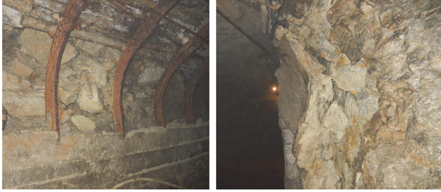
FIGURE 1: Existing supporting methods of broken rock mass.
