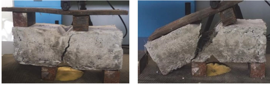
FIGURE 9: Crack pattern on specimens subjected to shear load.
