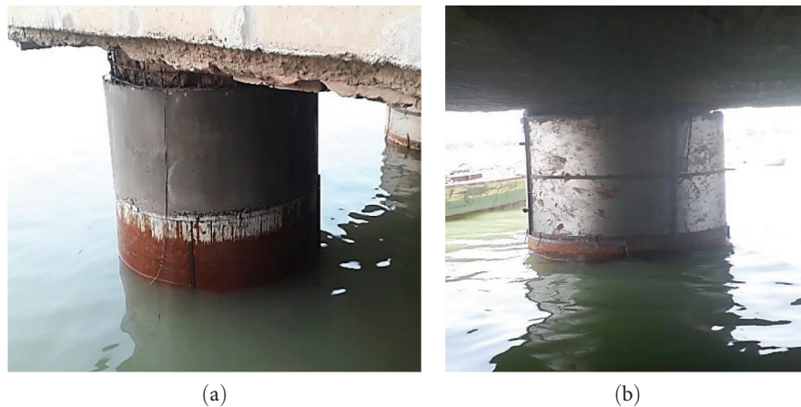
FIGURE 20: Piles after completion of retrofitting.
