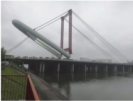
FIGURE 11: Process of rotation for tower.
