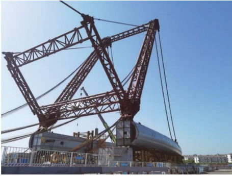
FIGURE 5: Rotation of chief strut by assistant strut.
