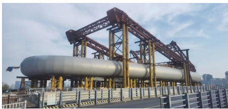
FIGURE 4: Preparing phase of chief strut and assistant strut.
