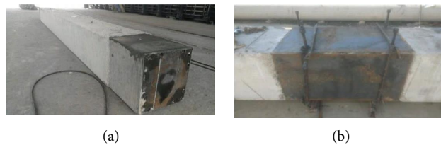
FIGURE 2: Scene diagram of precast concrete square pile. (a) Precast concrete square pile. (b) Precast concrete square connection pile.
