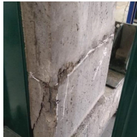
FIGURE 20: Precast wall panel—slender 1—failure.
