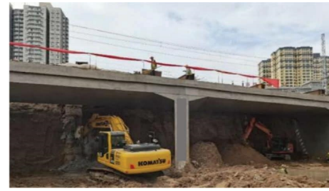
FIGURE 14: Xi'an Jingjiu road pipe-jacking tunnel engineering test site.
