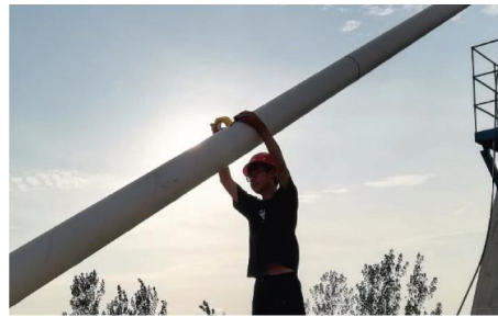
FIGURE 5: Field binding of cable force dynamic meter.
