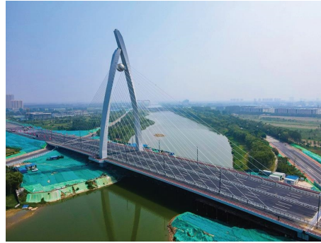
FIGURE 2: Actual project photos of Zhonghua Road Bridge in Liaocheng.
