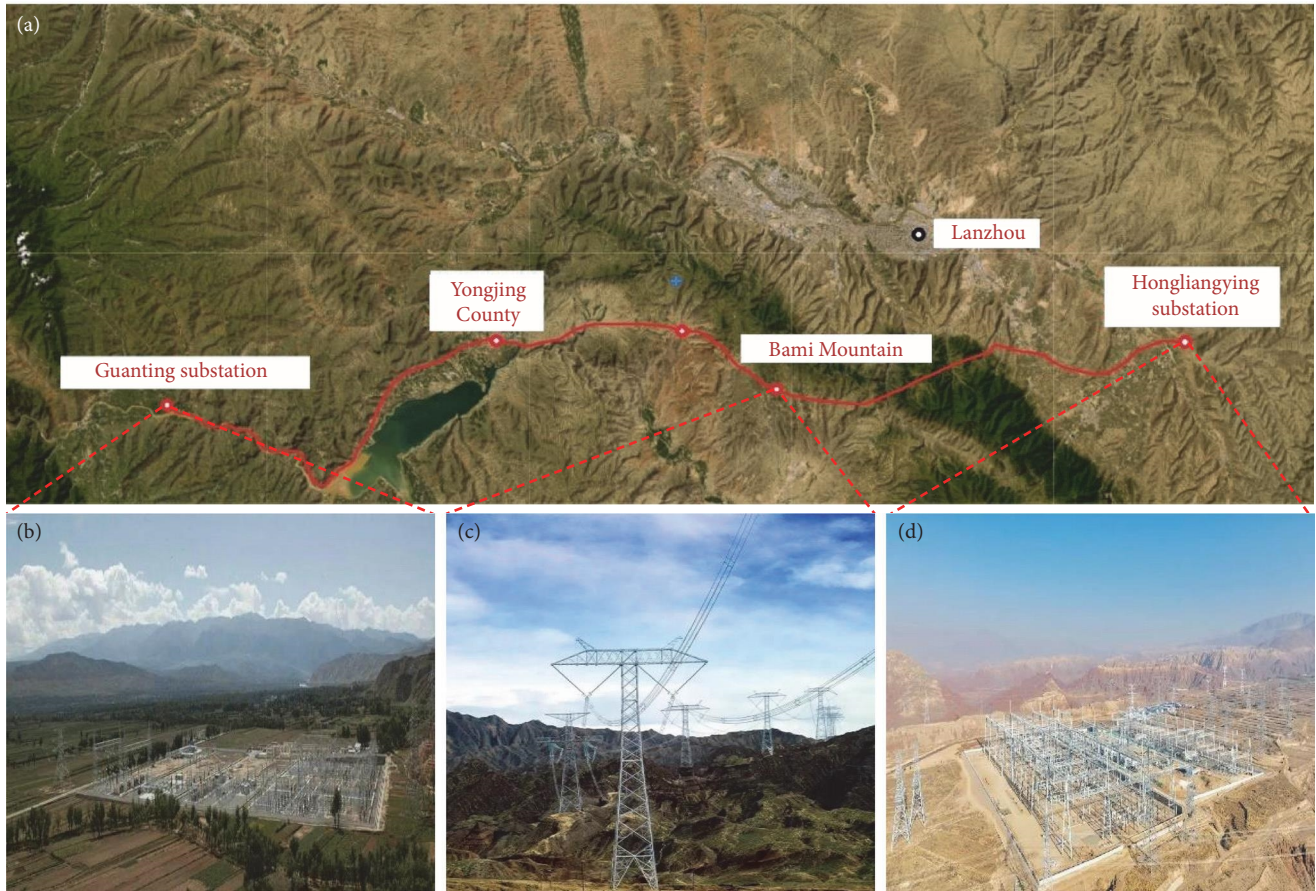
FIGURE 1: (a) Guanting–Lanzhou East electricity transmission line, (b) Guanting substation, (c) transmission tower, and (d) Hongliangying substation.
