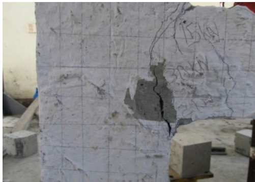
FIGURE 16: Failure pattern of CC specimen.
