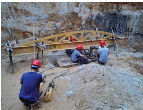
FIGURE 6: Reaction provided by the ground anchor.
