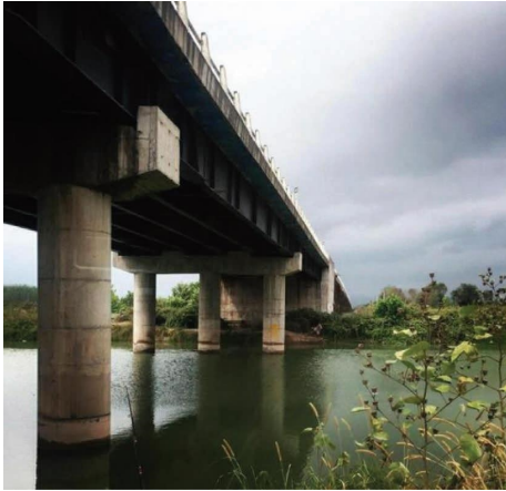
FIGURE 1: Concrete columns with a circular cross section in Guilan province in northern Iran.
