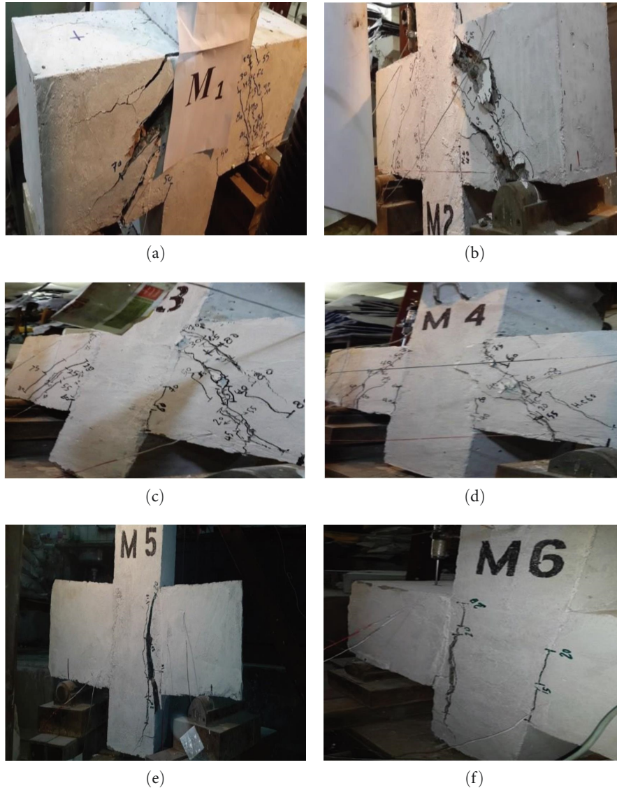
FIGURE 8: Failure modes of the tested specimens (note tested in inverted position).
