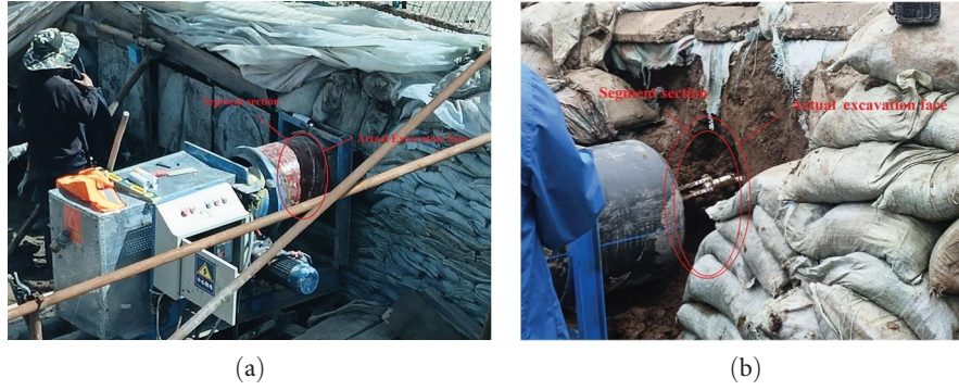
FIGURE 6: The construction difference between the two segments: (a) steel pipe segments and (b) PE tube segments.
