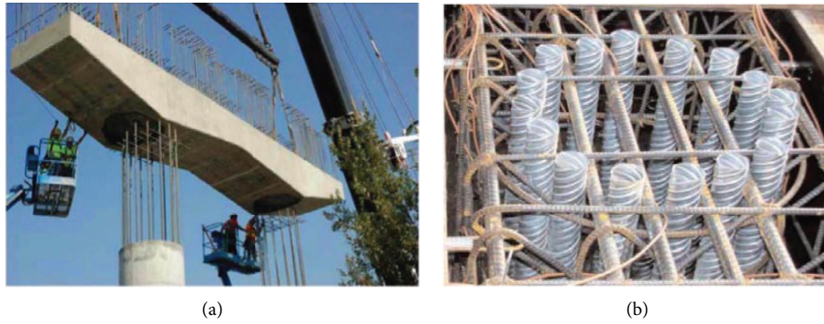
FIGURE 1: Prefabricated piers and columns connected with corrugated pipes [2]. (a) Prefabricated piers. (b) Corrugated pipes.
