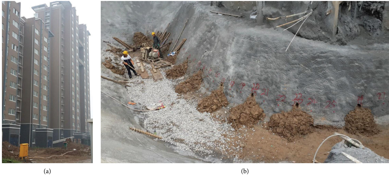
FIGURE 7: Underexcavation of case 1. (a) The building. (b) Underexcavation field.
