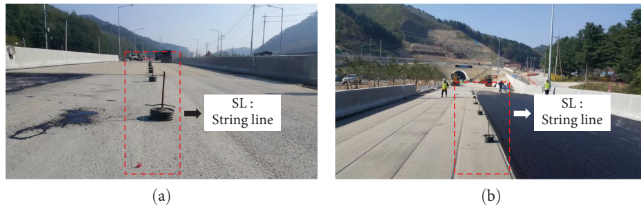
FIGURE 3: String-line (SL) system on a Korean expressway (Chuncheon-Yang Yang Highway, South Korea).
