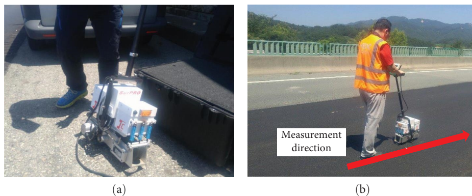
FIGURE 9: (a) IRI equipment and (b) IRI measurements.
