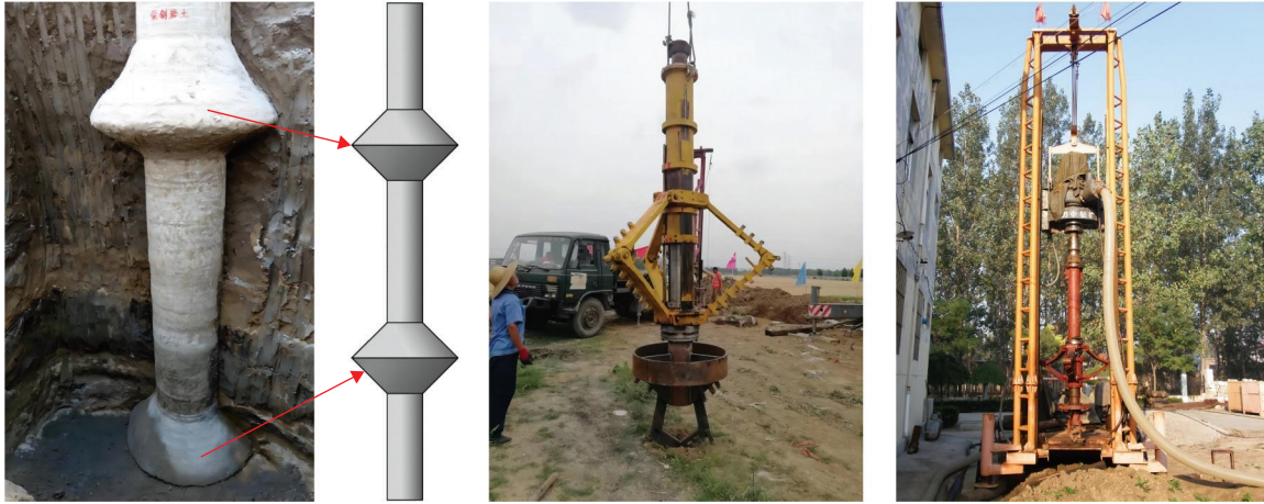
FIGURE 1: Schematic of NT-CEP pile and pile-forming machine.
