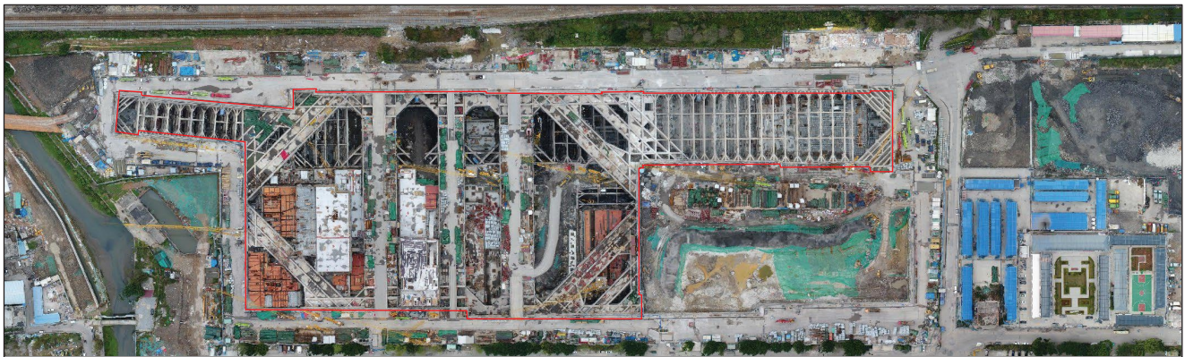
FIGURE 1: Schematic and layout map of the excavation: (a) shape and size of the excavation and (b) layout map of the excavation.
