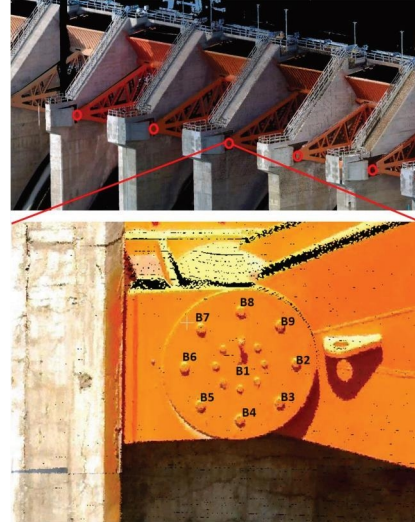
FIGURE 5: Zoom in of a trunnion gate and the nine measured bolts.
