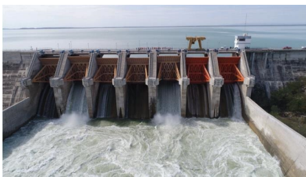
FIGURE 2: View of the reservoir, the control structure, and the buffer tank, as well as the embedding of the lateral abutments with the dam embankment.
