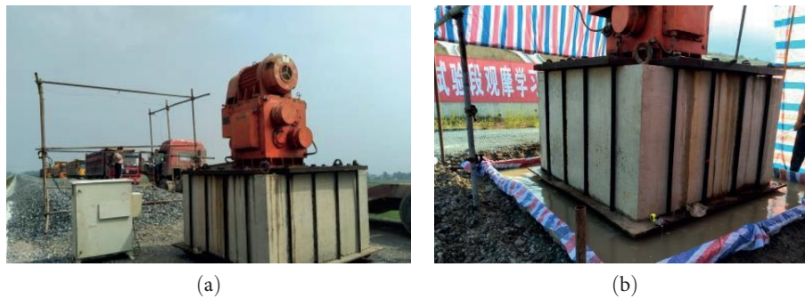
FIGURE 2: In situ vibration test. (a) ZBS60. (b) Infiltration simulation.
