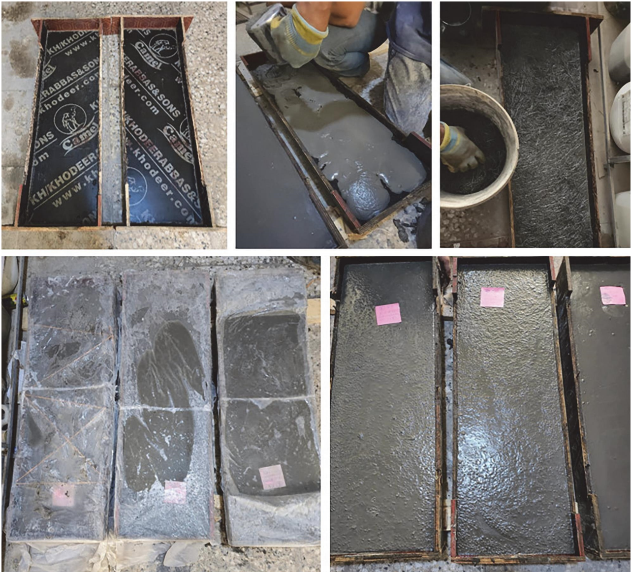
FIGURE 3: Casting of SIFCON plates.
