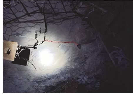
FIGURE 7: Cracking of the roof surface after blast roof cutting.
