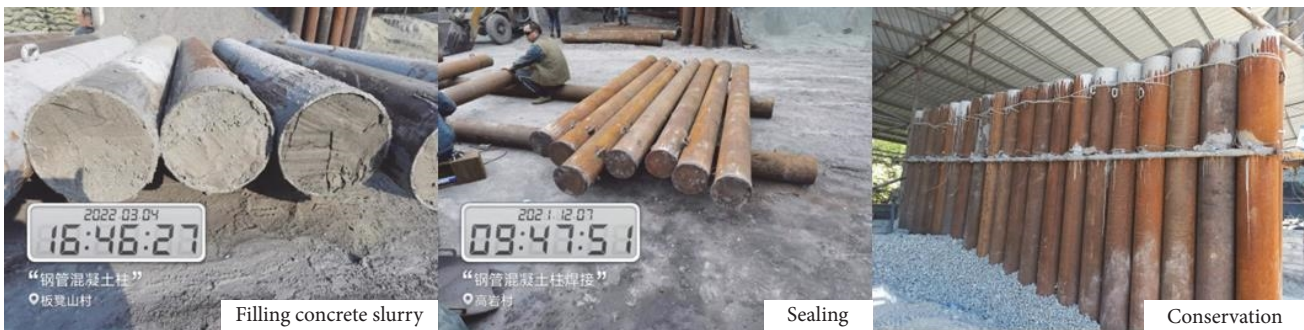
FIGURE 17: Preparation of steel pipe concrete columns.
