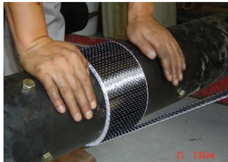
(a) Winding onto the rotating drum on one side
