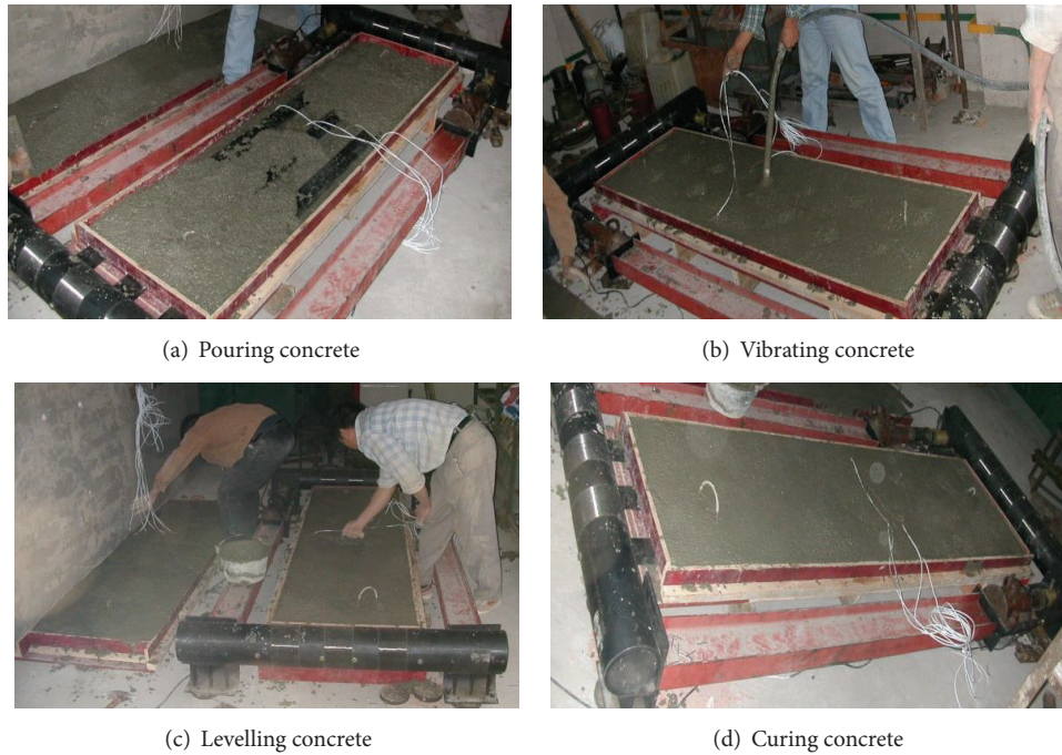
FIGURE 8: Construction process of the concrete slab.
