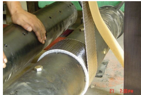
(b) Applying tension before unwinding
