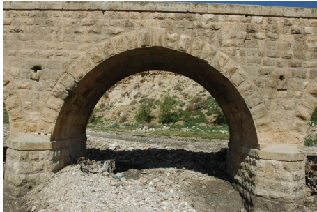
FIGURE 3: Elevation view of an arch and piers.
