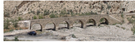
FIGURE 1: General view of the bridge.
