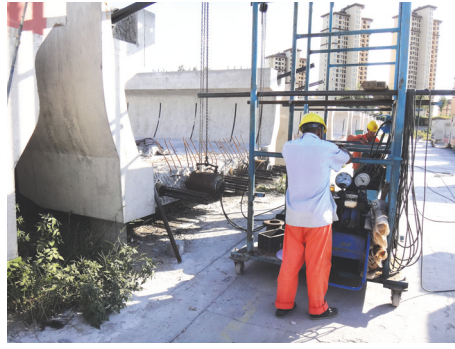
FIGURE 7: Posttensioning construction of U-shaped girder.
