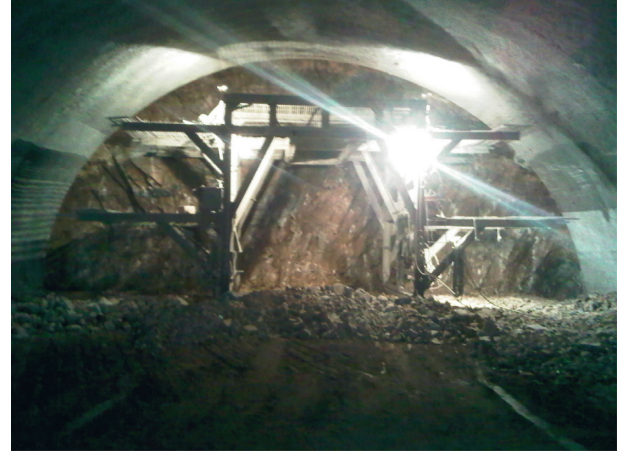
FIGURE 2: Picture of the Qixiaying tunnel.
