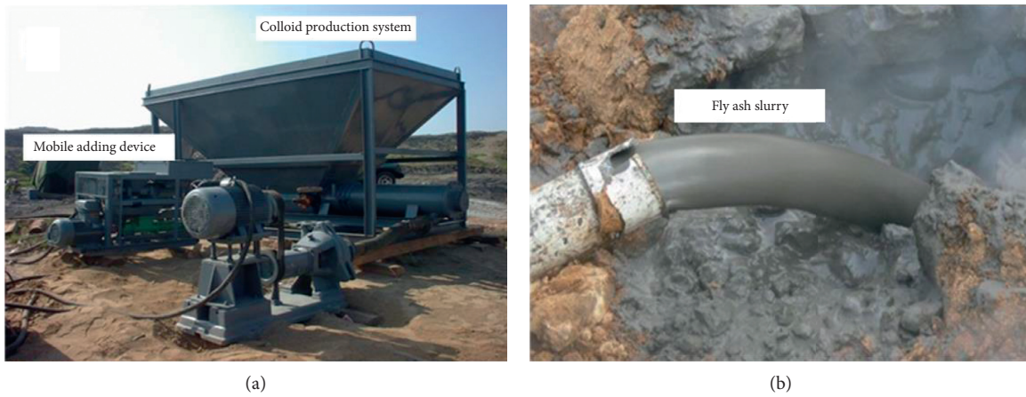
FIGURE 9: The application of fly ash slurry in the fire area.
