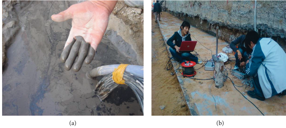
FIGURE 6: Test process. (a) Grouting. (b) Testing.
