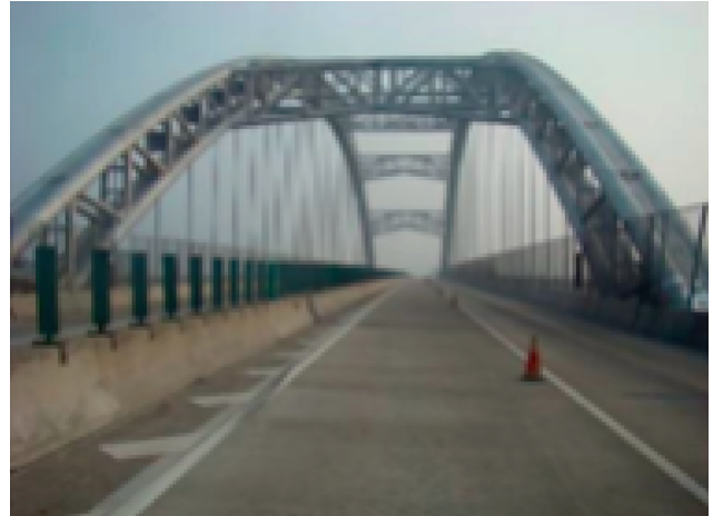
FIGURE 6: Liujing Yujiang superbridge.
