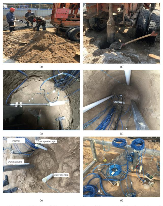
Figure 1: The field test. (a) Mixing lime soil. (b) Lime soil by using the hammer. (c) Sensor in the hole. (d) Sensor layout. (e) Layout plan of the pile top. (f) Test site after levelling.
