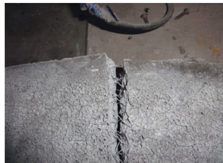
Wire meshes after cracking of the specimen
