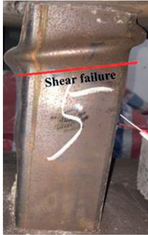
FIGURE 2: The shear failure of oblique circular bulge.
