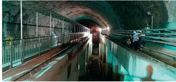
FIGURE 1: The field investigation in the tailrace surge chamber.
