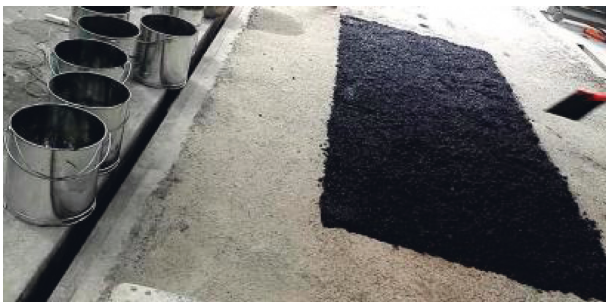
FIGURE 6: Paving the hard sandstone asphalt mixture.
