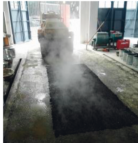
FIGURE 7: Compacting the hard sandstone asphalt mixture.
