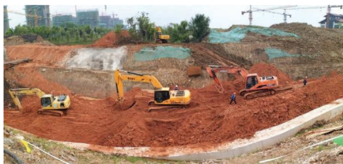
FIGURE 5: Excavation site of the river-crossing section.
