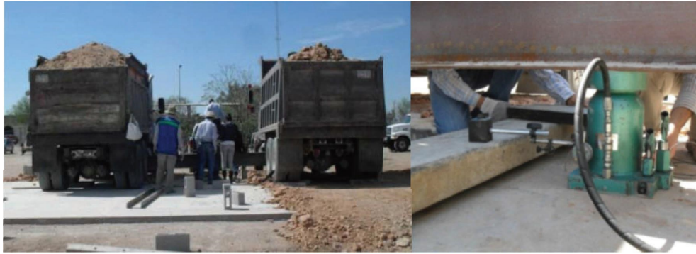
FIGURE 5: Field mounting for slab deformation.
