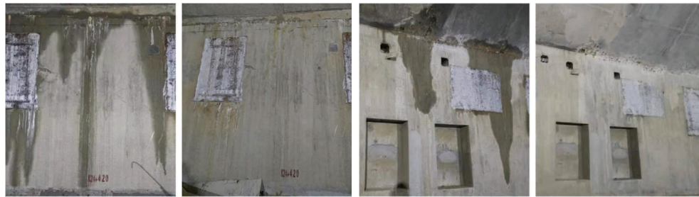
FIGURE 15: Inspection of the partial grouting effect.
