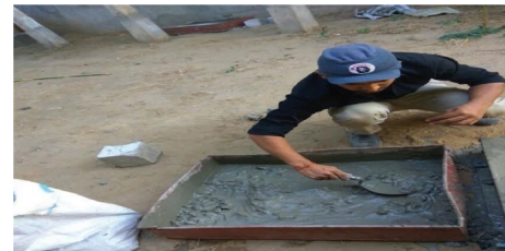
FIGURE 4: Preparation of concrete (source: author).
