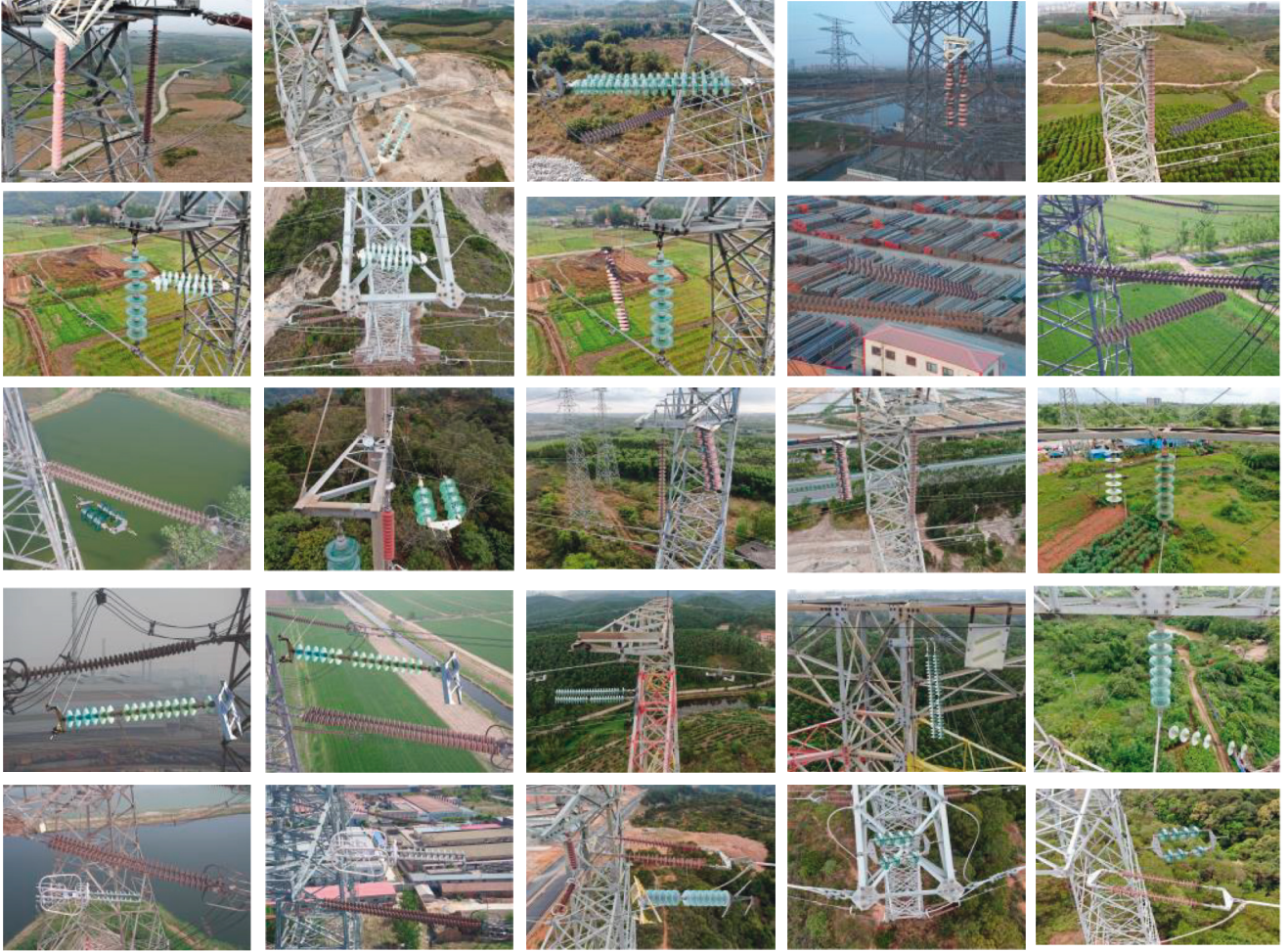
FIGURE 4: Parts of generated defective insulator images.
