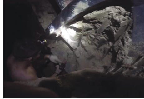
FIGURE 1: “Mud cake” at cutter head opening.
