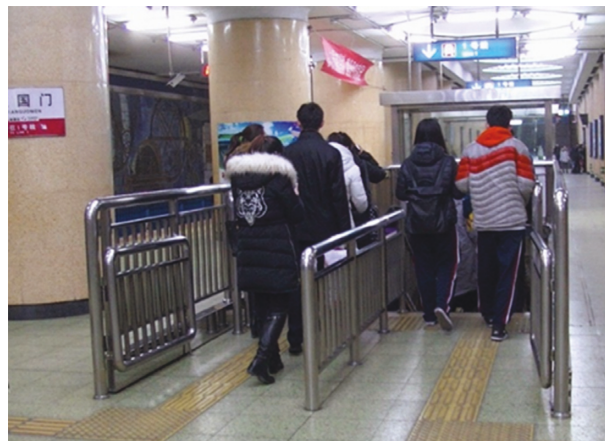
FIGURE 2: The guardrail in front of the escalator in Beijing subway station.
