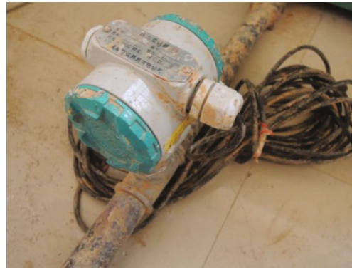
(b) Grouting pressure monitor
