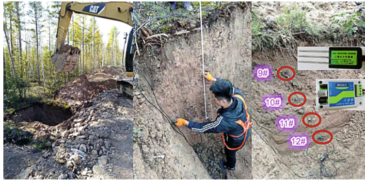
FIGURE 6: Construction glimpse of moisture sensors.
