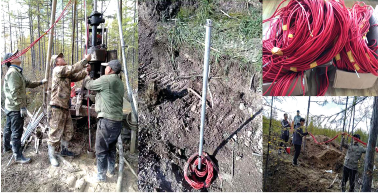
FIGURE 5: Construction glimpse of the temperature sensor.
