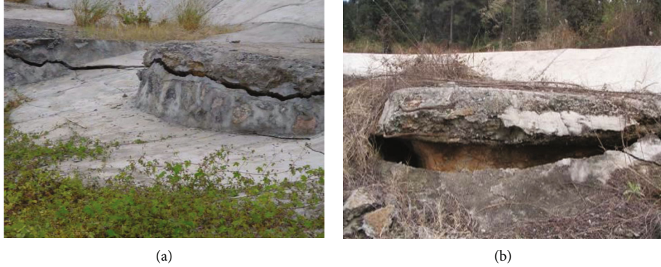
FIGURE 2: (a) Crack behind the piles of the third step in 2003. (b) Crack behind the piles of the third step in 2006.
